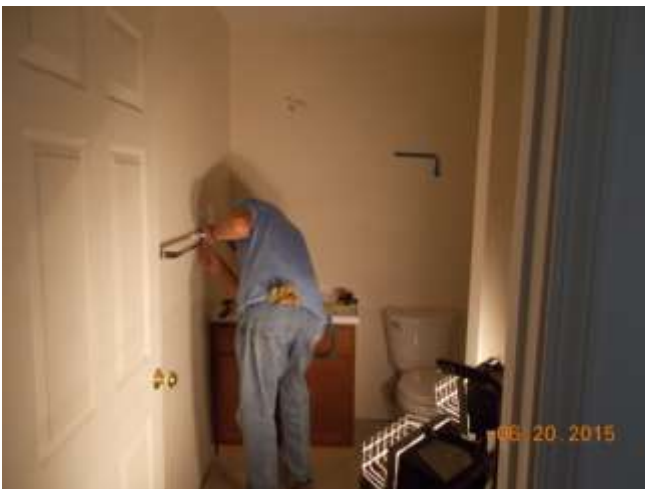
Hardware being installed
