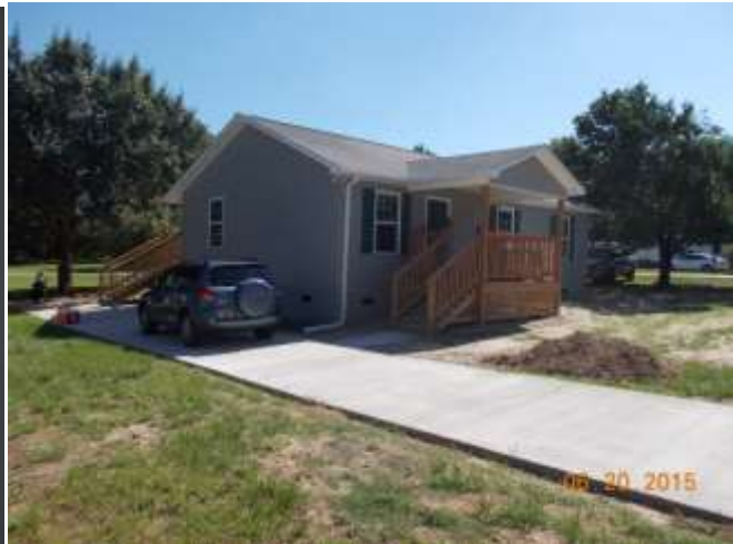
Driveway is complete
