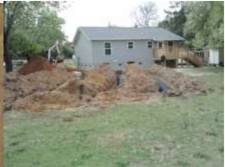
Septic system work in progress
