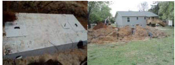
H & H Street septic system is now complete
