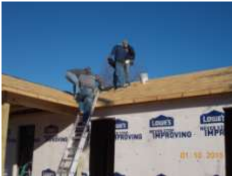
Work continues on a very cold day
