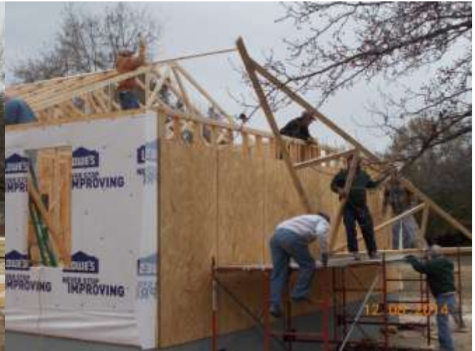
Tom Horn (on right) and other volunteers from Mount Vintage Plantation hoisting the roof joists on a cold Monday morning
