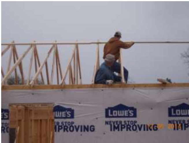
The roof supports being erected guided in place by Ben Hills
