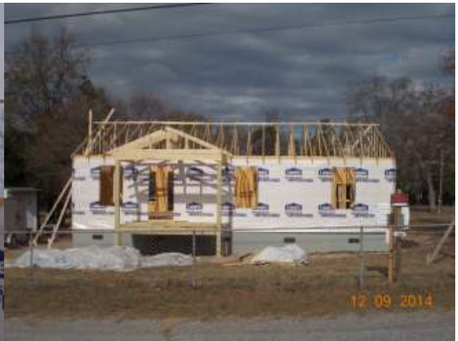
Roof supports and front porch ready for the next phase
